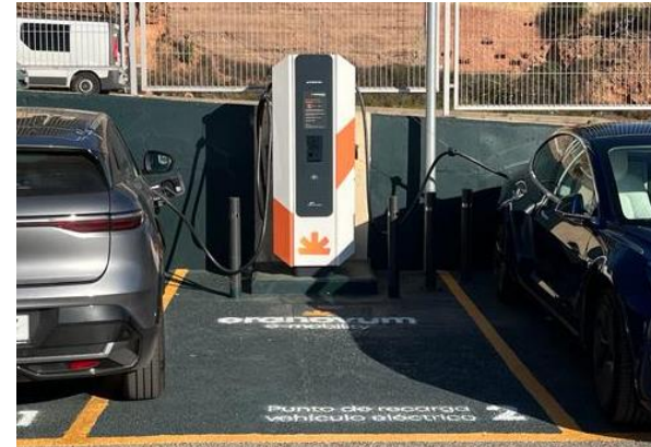
Serve our energy to our EV drivers
